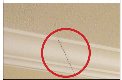
Interior trim crack
