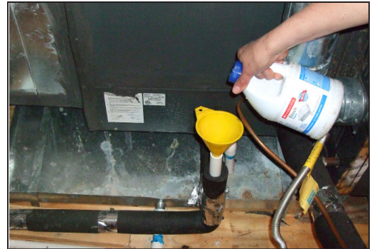
HVAC drain line by furnace in attic
