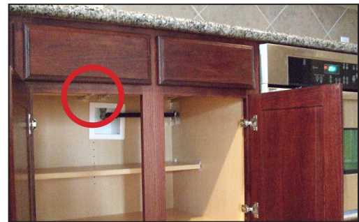
Gas shut off valve
