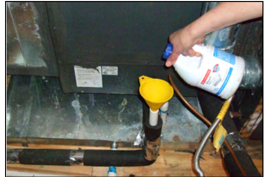
HVAC drain line by furnace in attic
