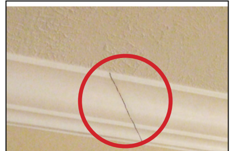
Interior trim crack
